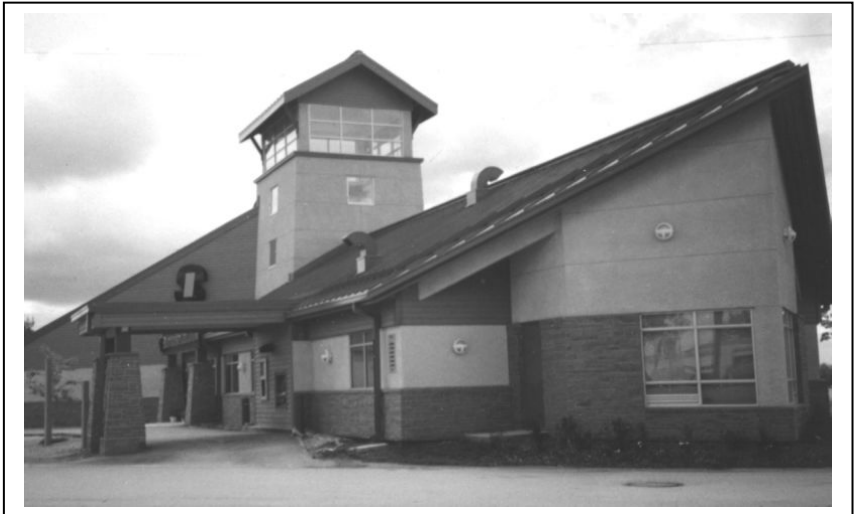
SICU's new building in Lac du Bonnet
